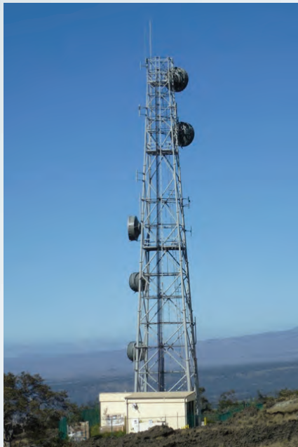
Ka'upulehu Radio Tower
