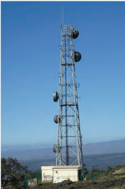
Ka'upulehu Radio Tower
